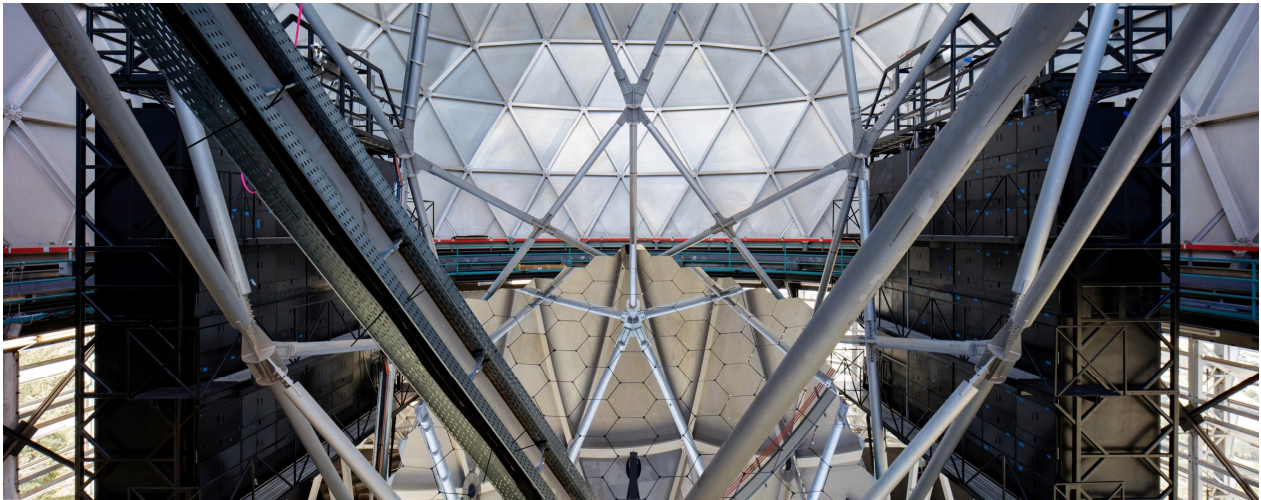
Figure 8: View of the HET from the front showing the primary mirror and the large VIRUS enclosures either side of the telescope structure. They sit on the VIRUS support structure (VSS), which moves on air bearings to follow the azimuth setting of the telescope. The phase separator tanks of the VIRUS Cryogenic System (VCS) can be seen mounted to the top of each enclosure.
